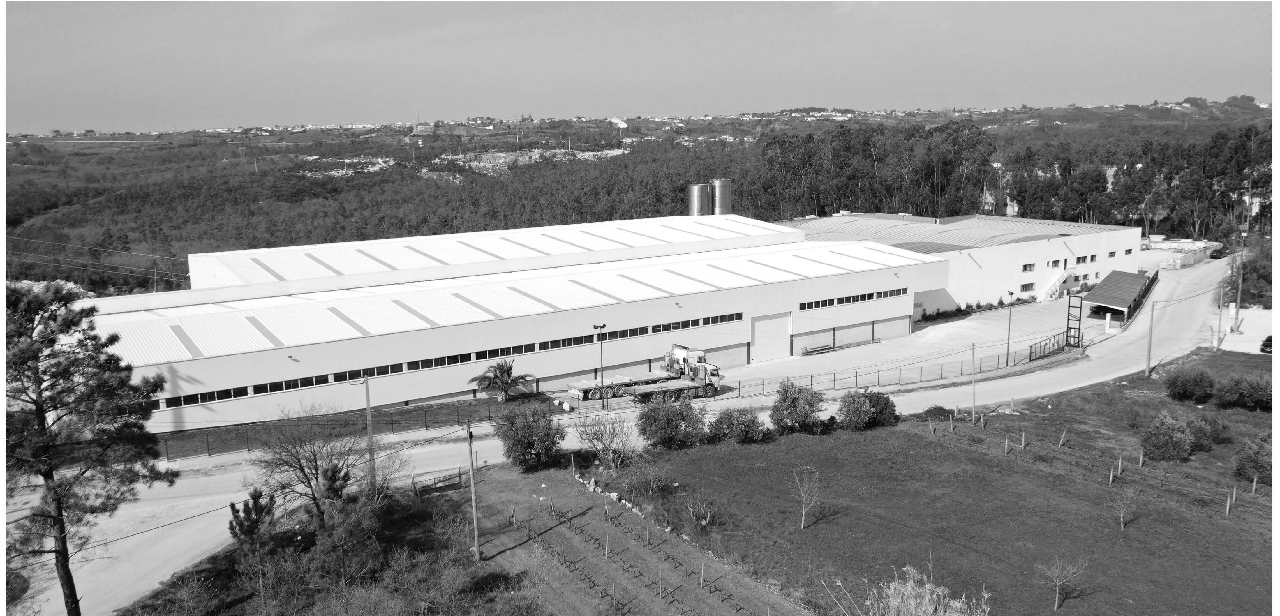
NEW FACTORY BUILDING
